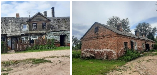
Fig. 15, 16. Villages Progress, Spartaks. Workers' house was adapted to a multi-apartment building in the post-war years [photos by A.Ziemeļniece, 2024]
