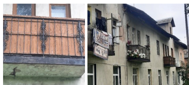
Fig. 8, 9. Village Progress. 2-multistory residential apartment buildings with balconies and ventilation windows [photos by A.Ziemeļniece, 2024]
