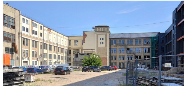
Fig. 2. Contemporary view of rubber factory "Kvadrāts" at Latgales iela 322/324 with additions from the 1970s and on-going process of functional and architectural conversion
