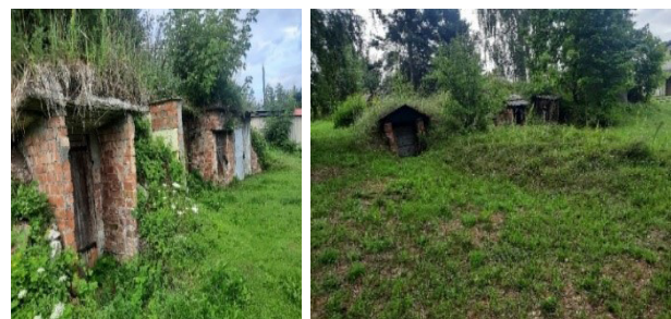
Fig. 4, 5. Villages Spartaks, Progress. Surface brick cellars with sod, 20th century, 50s [photos by A.Ziemeļniece, 2024]
