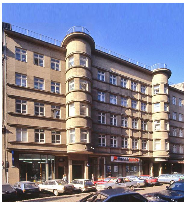
Fig. 11. Building of printing press "Rota" at Blaumaņa iela 38/40. Architect Alfrēds Birkhāns. 1934 [photo: Jānis Krastiņš]
