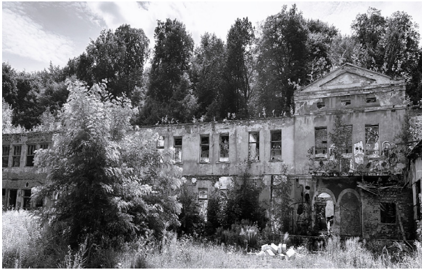
Fig. 2. The existing state of the main historical building, 2023 [photo by the authors]
