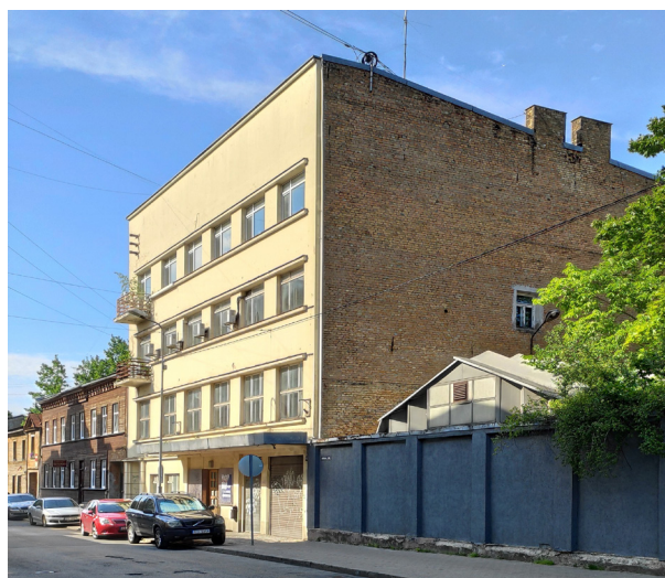
Fig. 5. Administrative building of the confectionery factory “V. Ķuze” at Artilērijas iela 55. Architect Aleksandrs Klinklāvs. 1934
