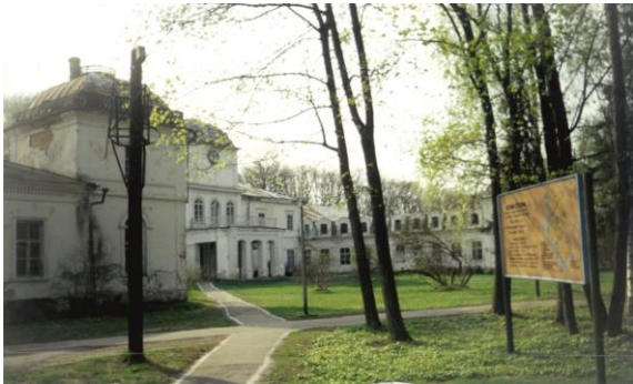
Fig. 7. View of the manor park of Khomutets [photo by L. Shevchenko, 2012]
