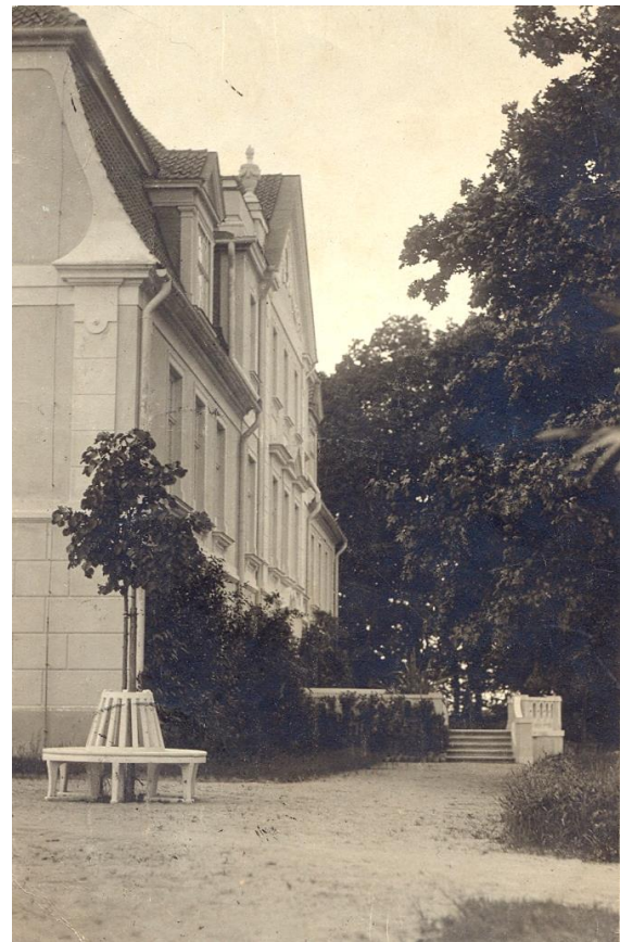
Fig. 11. View of Malpils Manor. Photo of 1930s [NKMP PDC]
