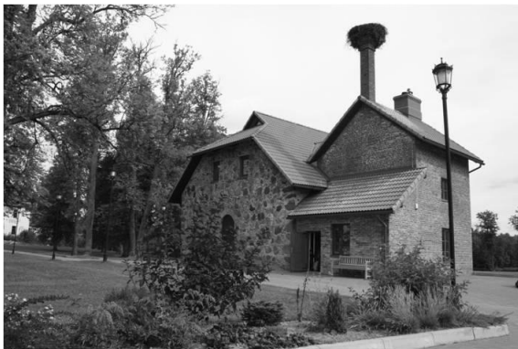
Fig. 8. The threshing barn with the drying-kiln [Source: photo by the author, 2009]
