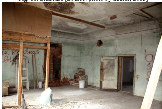
Fig. 11. The central room of the Smiltene rectory [Source: photo by author, 2015]
