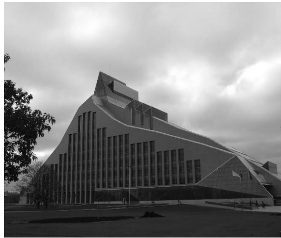
Fig. 7. A view of the NLL building from the side of the Daugava River [Source: photo by author private archive, 16.10.2014]
