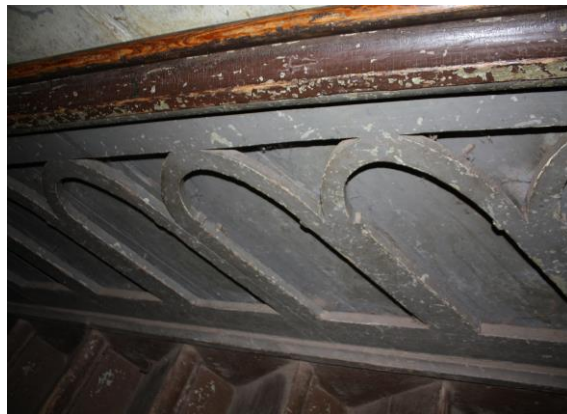
Fig. 10. Staircase [Source: photo by author, 2015]
