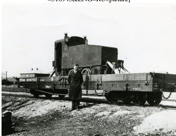
Fig. 7. Old rails at Pāvilosta [9]
