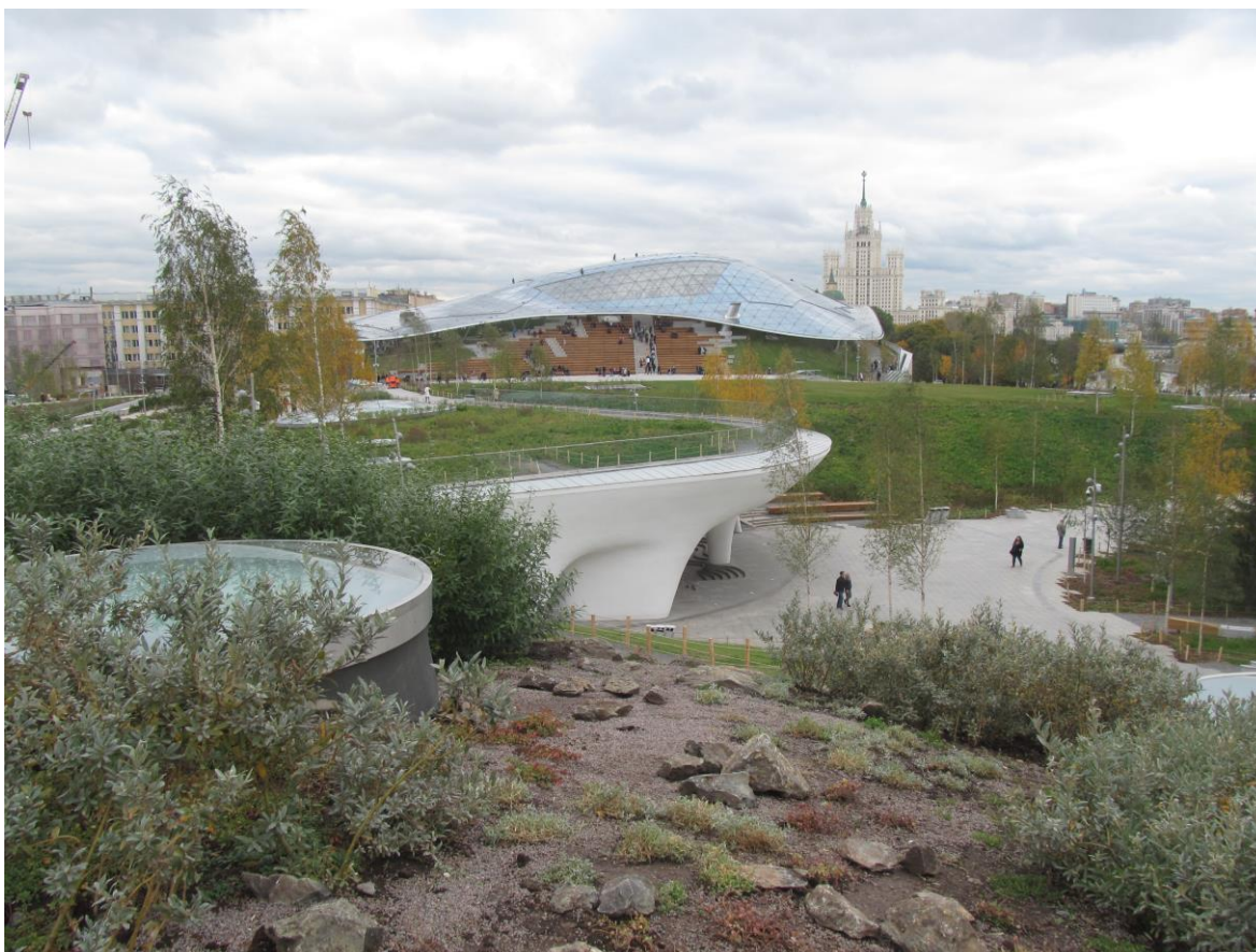
Fig. 9. A view of the "Reserve Embassy" and the "Glass Crust" [photo by the author]
