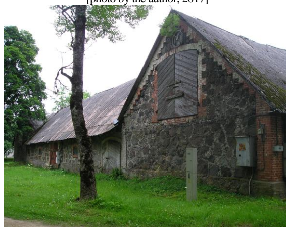
Fig. 6. Enclosure [photo by the author, 2017]
