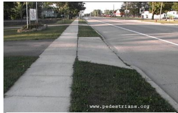
Fig. 5. The good solution for pedestrian way and driving way intersection on drive-ins to urban quarters, open areas and courtyards Source: www.pedestrians.org [online 4.08.2018].
