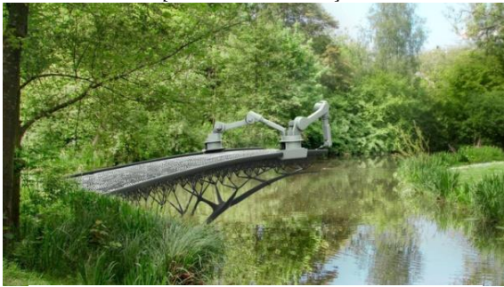
Fig. 6. 3D printed pedestrian bridge. Amsterdam. 2016.
