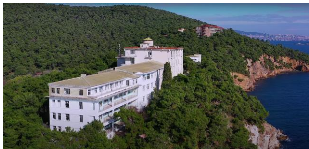
Fig. 3. The Sanatorium in the first location - Location A on the map [21]
