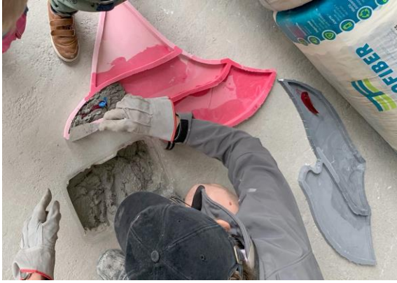
Fig. 7. Casting first floor pieces in standard gray concrete [photo Arne Riekstins, 2021]
