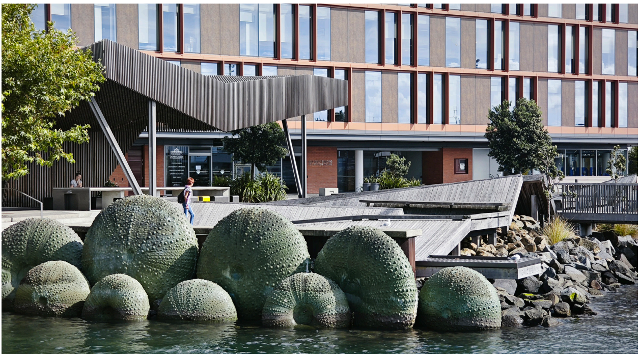
Fig. 3. The folded plane: deck surface stepping to form seating and viewing terrace without change of material. The section, rather than an added object, produces the sitting edge [photo by the authors, 2026]
