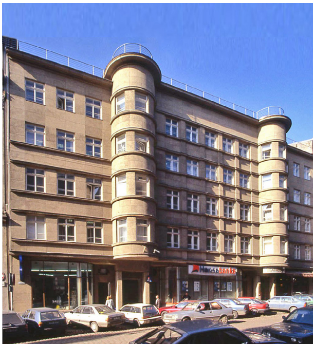
Fig. 11. Building of printing press "Rota" at Blaumaņa iela 38/40. Architect Alfrēds Birkhāns. 1934 [photo: Jānis Krastiņš]
