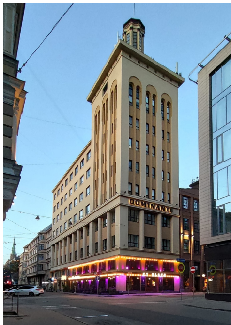
Fig. 12. Building of printing press of joint stock company "Riti" and newspaper "Segodnya" at Dzirnavu iela 57. Architect Alfrēds Birkhāns. 1939
