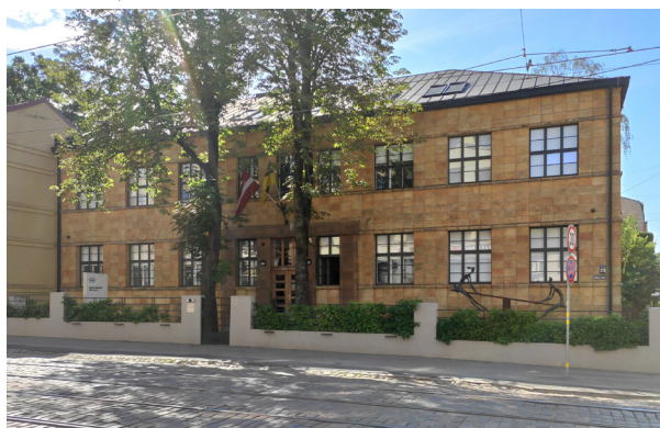
Fig. 14. Office building of "F. Hoffmann–La Roche" at Miera iela 25. Architect Aleksandrs Klinklāvs. 1931
