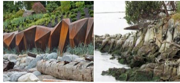
Fig. 10. The corten steel retaining wall compared to Saturna Island sandstone formations [Photo© Left: Tim Swanky, Right: Paul Sangha Landscape Architecture]
